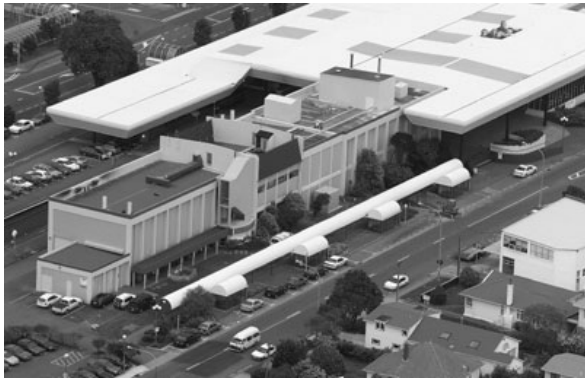
A Wellington water treatment plant, now managed with Derceto
