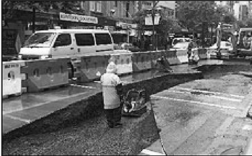
Figure 1: The Auckland CBD was subject to extensive digging operations as TelstraSaturn and other operators laid ducts to carry their new fibre optic networks.
